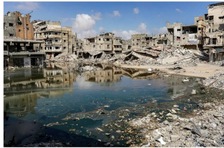
Sewage water from collapsed underground pipes covers an area by destroyed buildings in Khan Younis in the southern Gaza Strip on July 8, 2024. (Photo by BASMAH TALEBAFF via Getty)
